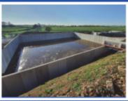
to 3.7m, siliage with 10t vehicle surcharge to 3.2m and earth to 3.4m depths. 145mm panels can be also be used if retained heights are reduced by 0.3m to 0.4m depending on retained material
